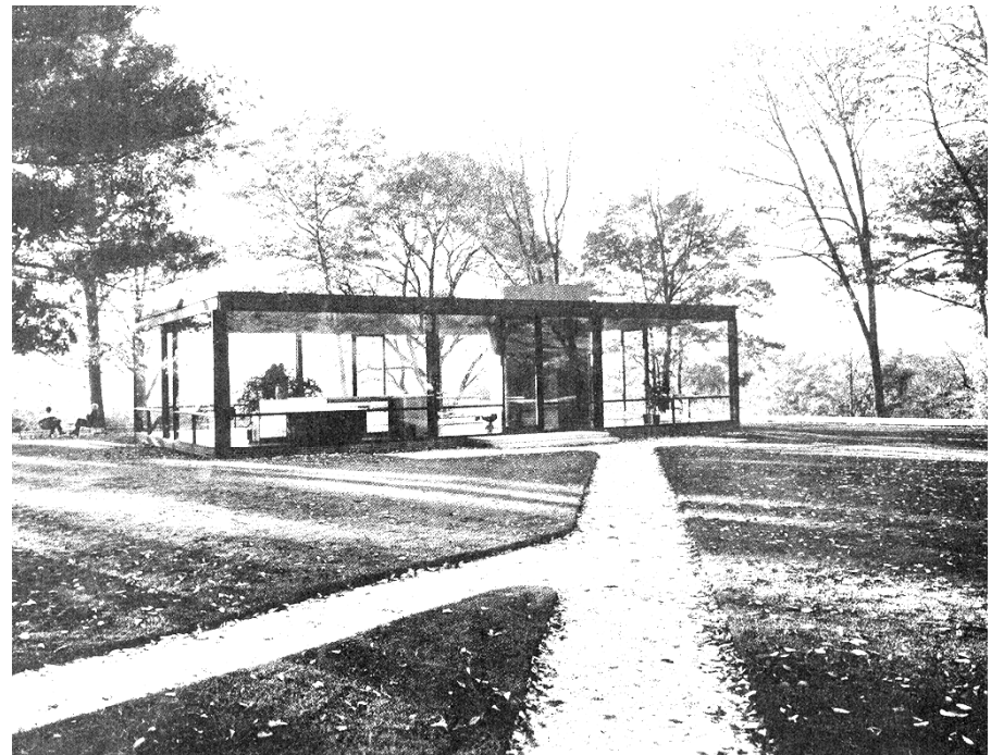
Glass House, New Canaan, Connecticut, 1949, Philip Johnson
